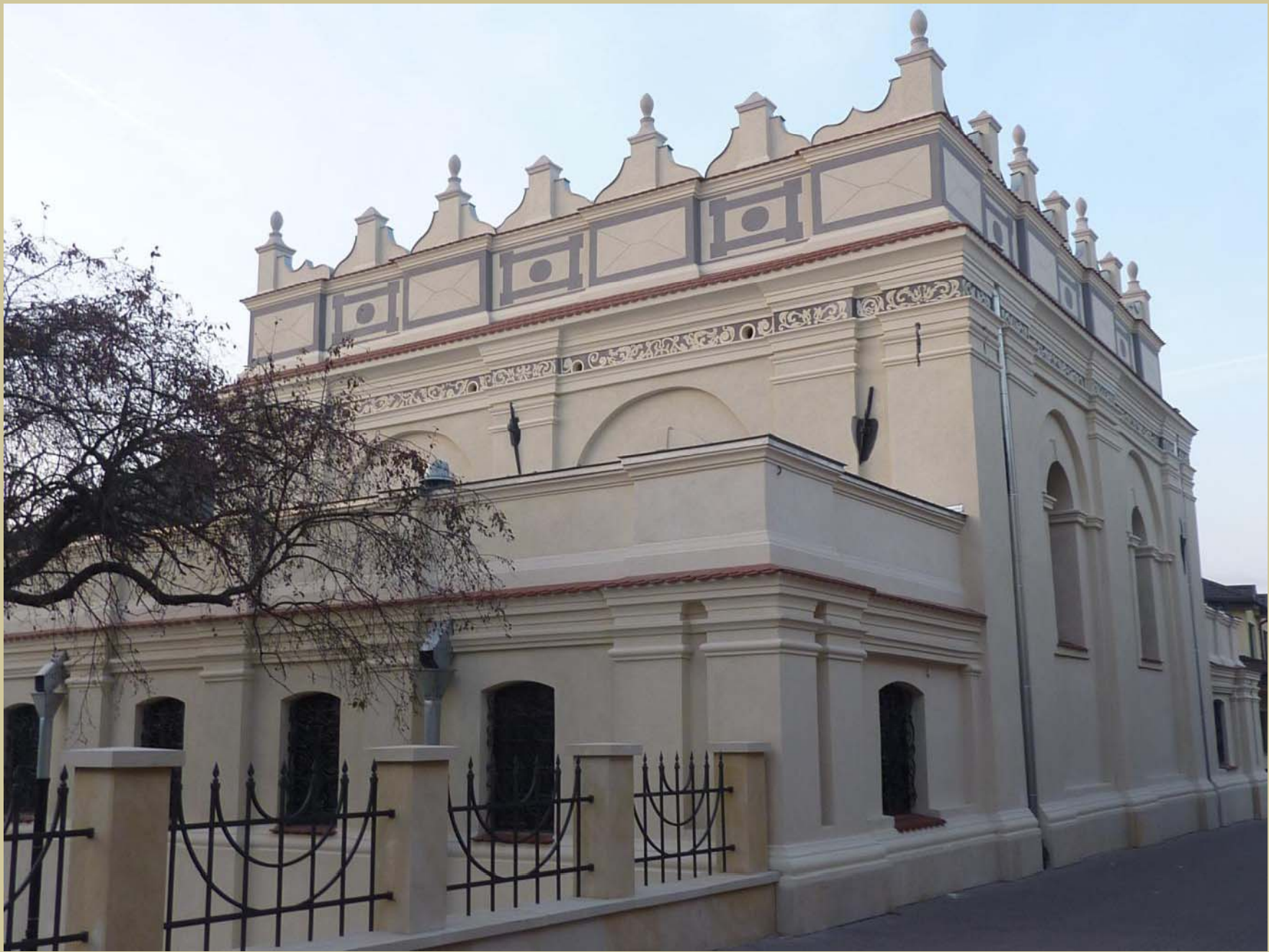
Synagogue in Zamość; general renovation July 2009 - summer 2010
